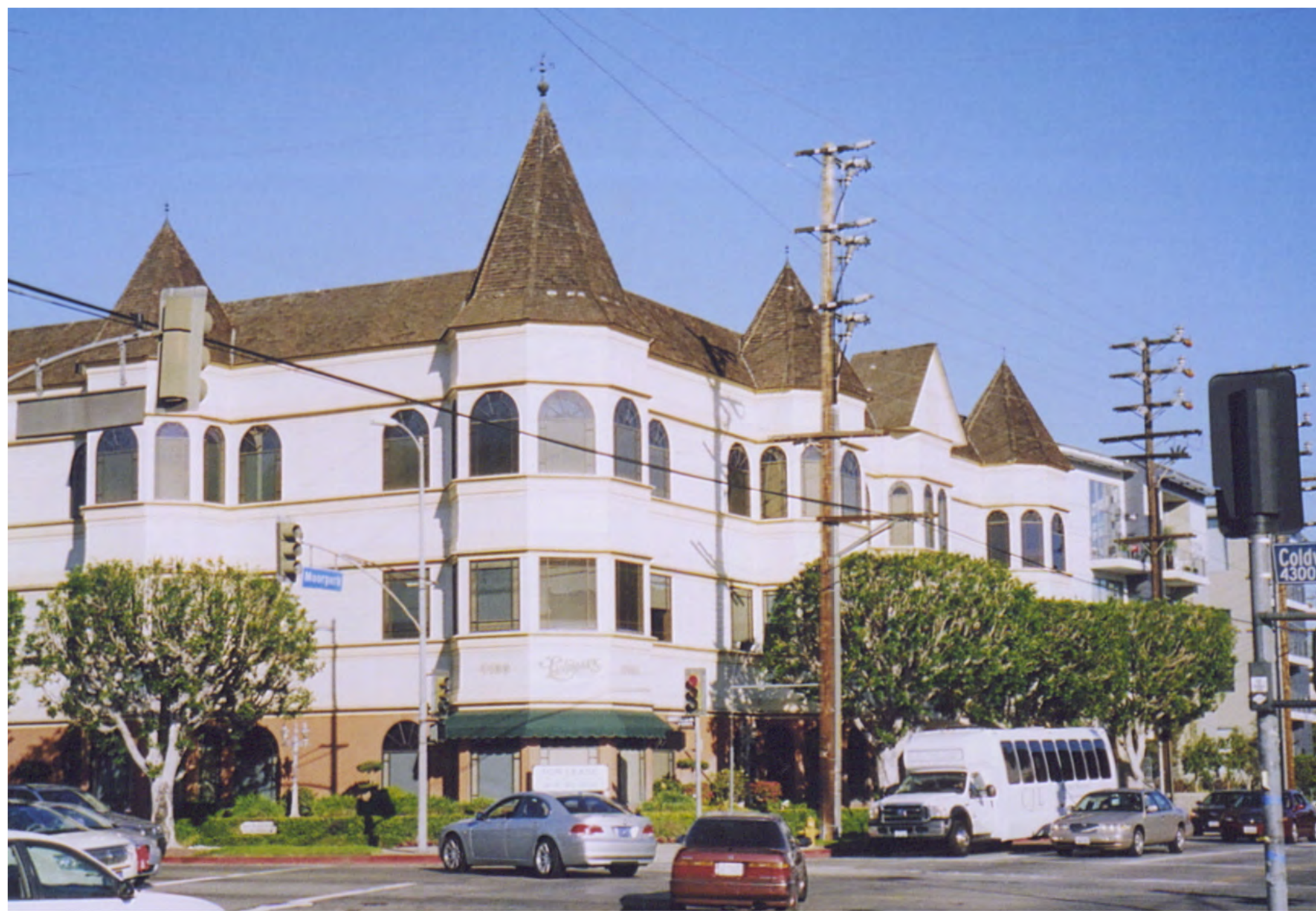
This mid-rise office building has a sloped roof, portions of its facade that extend outward with bay windows and steep, pointed roofs above the bay windows that extend further above the roofline. These features result in the building having a Victorian architectural style which is rare for the Valley and results in it having a high level of architectural quality.
